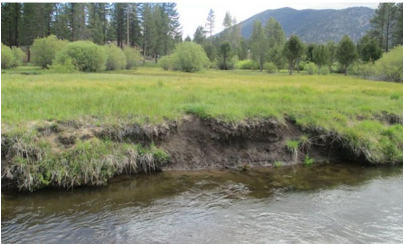
Figure 15. G Channel erosion
