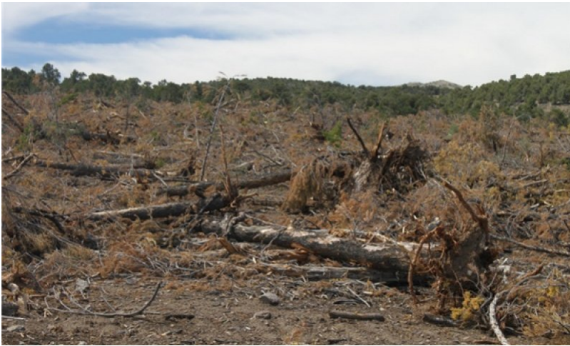
Figure 13. Tree Removal_P. Novak-Echenique_7/2012
