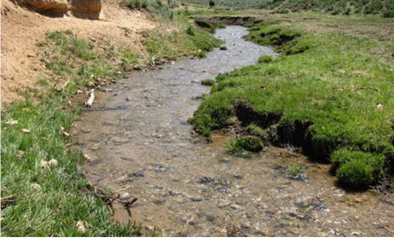
Figure 15. Bank sloughing and channel widening
