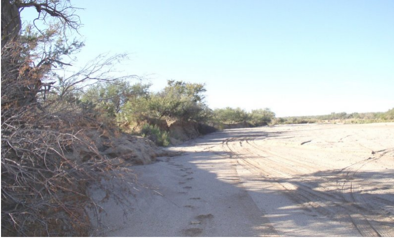
Figure 7. Sandy Bottom 12-16" pz, eroded
