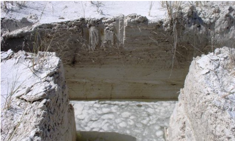
Figure 6. Transformer Soil Pit
