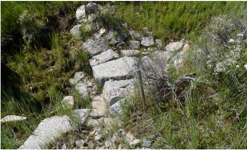
Figure 10. New rock work at headcut
