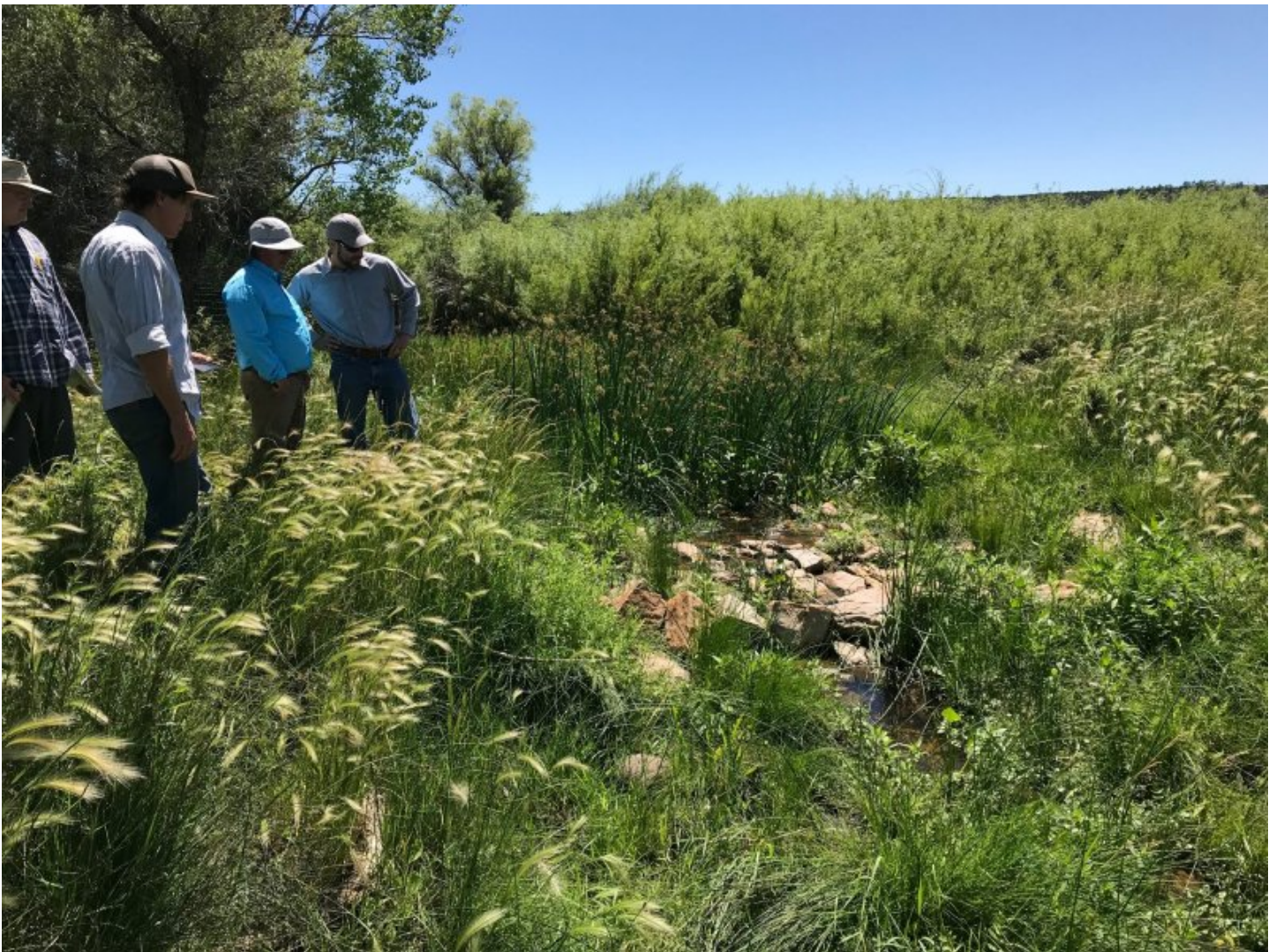
Figure 7. Riparian restoration along a section of formerly incised channel in the form of grade control structures such as 1-rock dams. Intended to reconnect parts of the floodplain to the water table.
