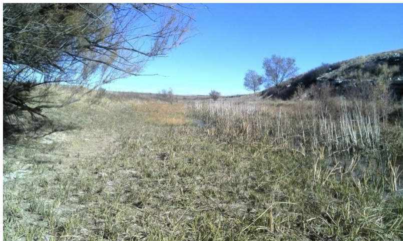
Figure 8. Active channel (2.1AC). Destabilization of the banks has widened the channel causing a high width to depth ratio, which is an unstable parameter for resisting further erosion during flood events.
