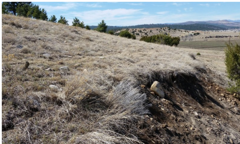
Figure 6. Community 1.1 on the riser of a strath terrace in San Miguel County, March 2017. State 1 occurs on the vegetated terrain above the cut. Note the thick topsoil exposed in the cut, and the grass-dominated plant community above.
