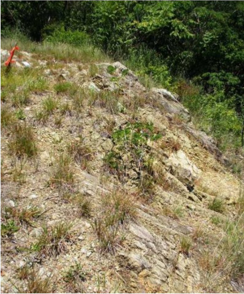
Figure 19. Excavated serpentine barrens, VanDuzer and Grymes Hill
