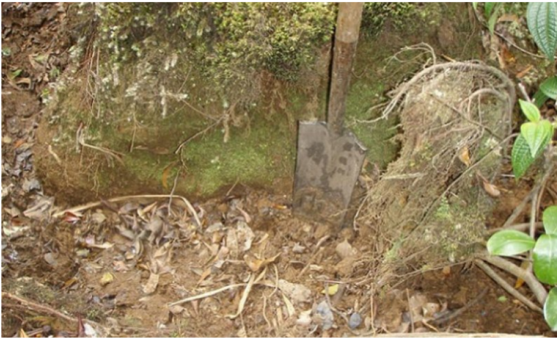
Figure 16. Closeup of erosion-caused pedestal 7/1/08 D Clausnitzer MU 905
